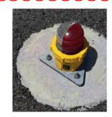
MID RANGE LIGHTING INSTALLATION. LED FITTING. CONCRETE FOUNDATION, FAA STYLE SERIES ISOLATION TRANSFORMERS INSTALLED IN SEPARATE ELECTRICAL PIT. SINGLE OR DUAL PRIMARY CABLES INSTALLED IN ONE
