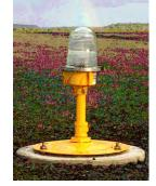
TOP OF THE RANGE LIGHTING INSTALLATION. GLASS LENS AND METAL BASE MOUNTED ON CONCRETE BLOCK WITH FAA STYLE BASE PLATE. DUAL PIT AND DUCT SYSTEM TO PROVIDE TOTAL SEGREGATION BETWEEN
