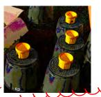
LIGHTS CAN BE MOUNTED ONTO PLASTIC VALVE BOXES. LIDS TEND TO BECOME BRITTLE AFTER 15 YEARS AND WILL PROGRESSIVELY NEED CHANGING, GOOD
